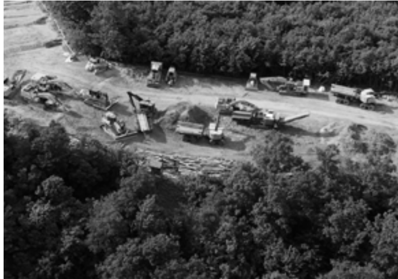
Construction on the Mountain Valley Pipeline.
