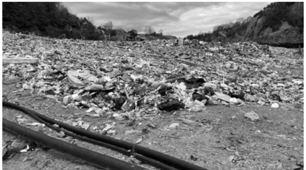
Inadequate cover and large working face at the Bristol, Virginia, landfill, as cited in the Virginia DEQ report detailing the April 21, 2022 onsite inspection. The quarry walls, seen along the sides, serve to direct stormwater into the landfill. Water mixed with the trash results in accelerated decomposition, elevated temperatures and increased gas emissions (photo courtesy of Virginia Department of Environmental Quality).
