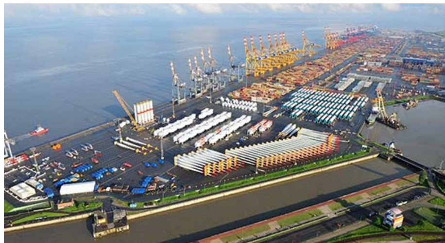
Pictured here is the OSW staging area in Bremerhaven Germany.
